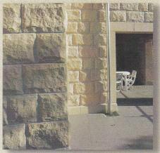
Numerous different moulds are used in production to ensure a wide variety of surface impressions and an authentic "handcut" look.
